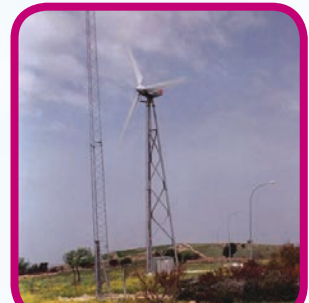
Al-Ibrahimiyyah Wind Farm
